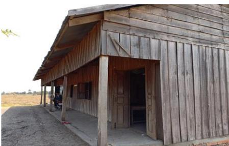
The wooden pillars supporting the structure are crumbling and could collapse anytime.
