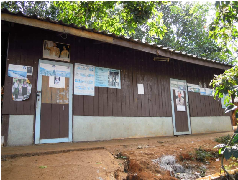
One of the two school buildings at CLC Community Learning Centre Tomato Village.
